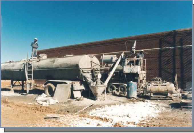
Workers pump lightweight insulating concrete to roof deck.
