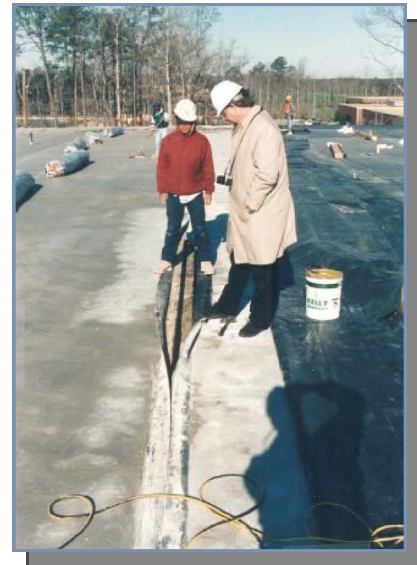
Inspector notes water-saturation under loose-laid 2001 EPDM sheet.
