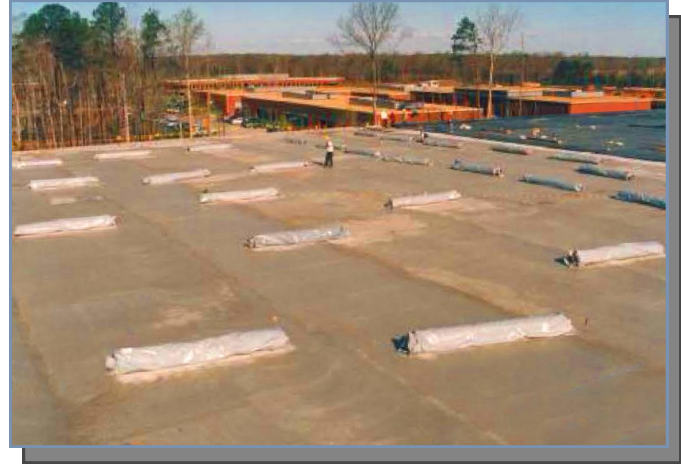
EPDM rolls placed upon deck surface saturated by heavy rains.
