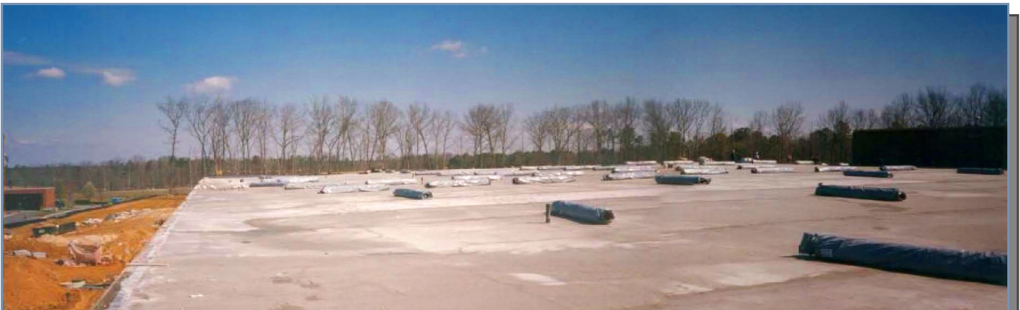
Rolls of 90 MIL EPDM in position to be loose-laid upon lightweight insulating concrete.
