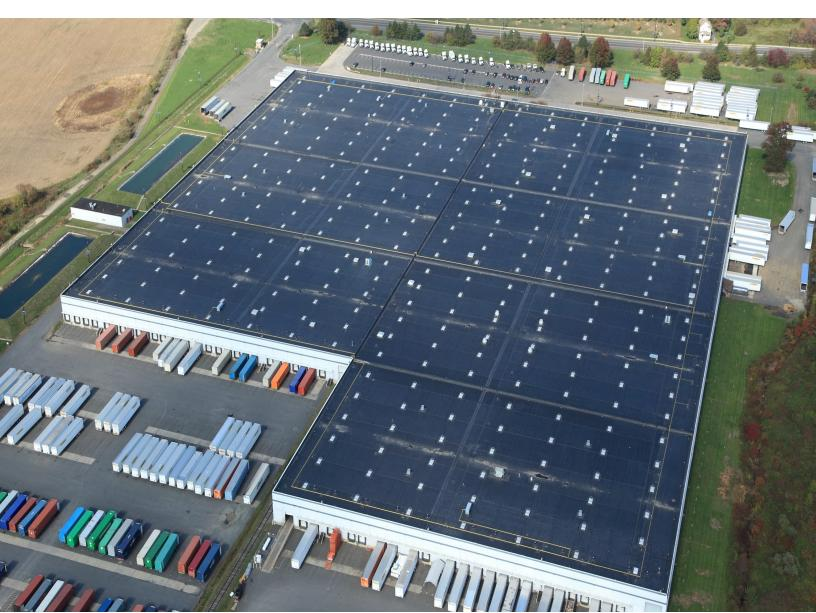
IN 1998 A 2001 COMPANY WIND VENTED ROOF WAS INSTALLED AT 66 CRANBURY STATION ROAD IN CRANBURY, NEW JERSEY. 822,000 S/F OF 45 MIL EPDM WAS THE ROOF MEMBRANE USED.
