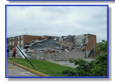
The walls of the gymnasium imploded and the roof deck failed. Yet, the 2001 WVRS membrane remained attached without adhesives, or mechanical fasteners.
