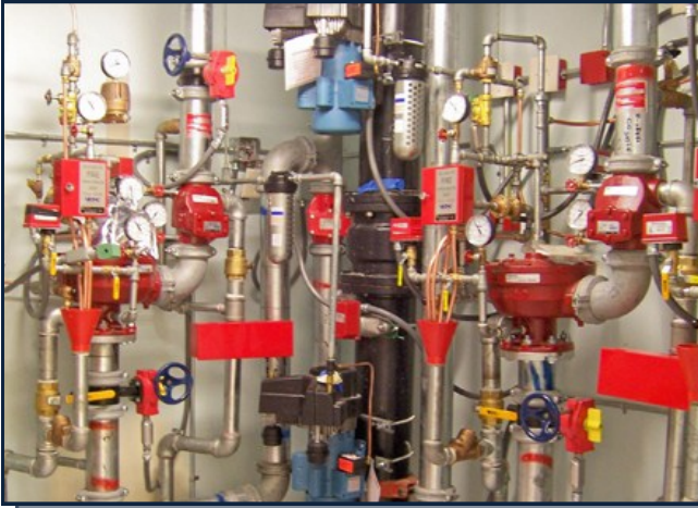
Data Center's Praction Valve Room
